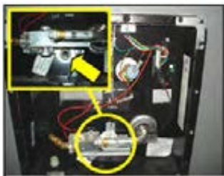
Water heater drain plug location
