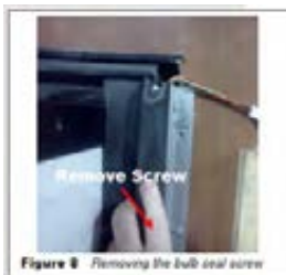
Figure 8 Removing the bulb seal screw
